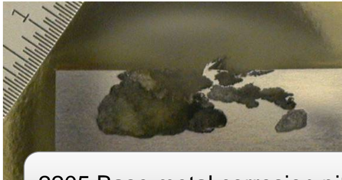
2205 Base metal corrosion pit after ~11 months of service
